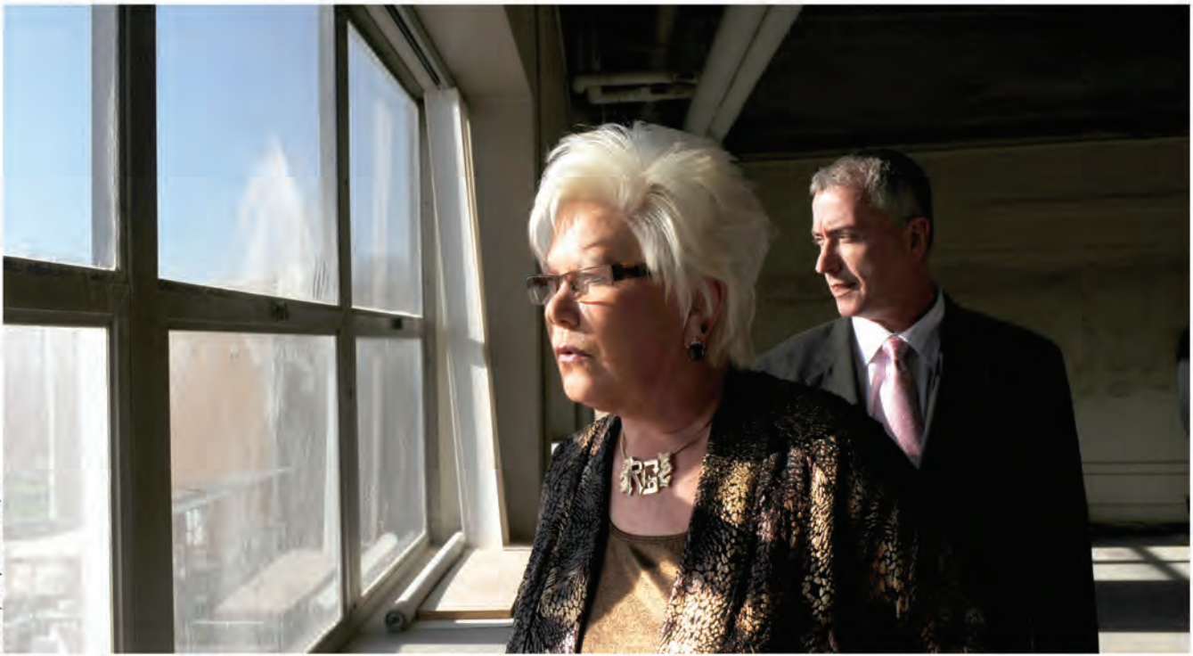
Roe Green (left) and College of the Arts Interim Dean Dr. John R. Crawford view construction of the Roe Green Center.
